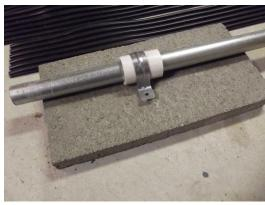
The edge framework can be clamped to the concrete pads with pipe/conduit via a sleeve of 1.5" pipe. The two hole pipe clamp and pipe sleeve can simply be glued to the concrete pad using Loctite PL Premium 3x construction mastic as the last step. This loose sleeve connection provides some flexibility in positioning relative to the uneven roof surface. These chain link fence top rails can also be bent to follow the roof shape.
