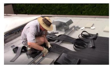
Use a chalk line and/ or the 2 lengths of Unistrut to mark the cuts on the fin tubes 5" apart. Cut the longer fin tubes first and attach those manifolds first. Then fold these out of the way before cutting the shorter fin tubes and attaching those manifolds. This way you can't make a mistake and cut a long fin tube short or glue a header to the wrong fin tube.
