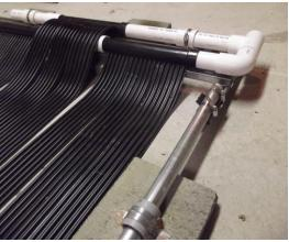
The Unistrut lengths are separated by a distance of 5" center to center or to match the spacing created by the tee and elbow at the corner where water enters or exits. If plumbing is 2" use a 2" tee, bushing and a 1.5" elbow.
