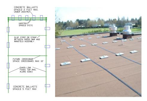
Glue strips are made of 2 tube wide Powerstrip fin tubing.
