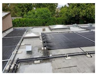
Fin tubes are flexible so they can be arranged to avoid roof obstructions and you can even curve the system to fit unusually shaped roofs.
