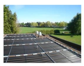
Cross members should be spaced about 10 feet starting from the manifold assemblies. One inch rigid conduit 2 hole or 1 hole pipe clamps with #20 all SS hose clamps can lock the cross members in place. The cross bars sit exactly on top the fin tubing and serve to hold the solar collector down just like a big strap right across it but stiffer.
