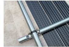
CROSS RAIL TO EDGE RAIL - SHORT STRAP AND 2) #20 ALL SS GEAR CLAMPS
