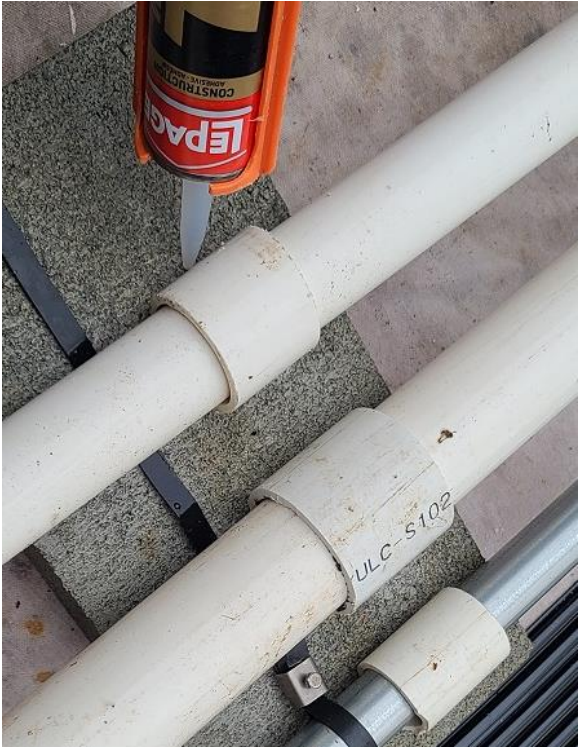
Slip collars glued to ballasts (flat roofs)
