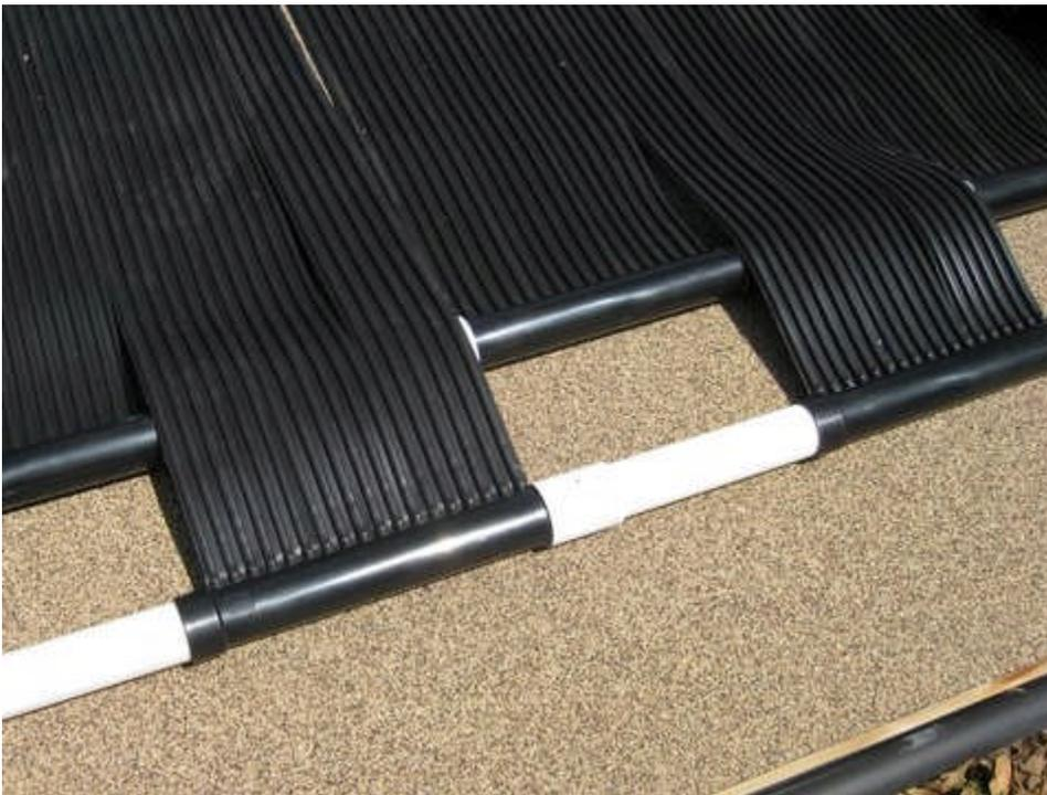
Note that with this technique we also eliminate the need for removable couplings. You have about 9.5 inches of pvc pipe between each headers so if you ever needed to replace one you'd simple cut the pipe and re-connect with a pvc coupling. You'll need a 1.5"
