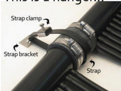
Note there are no removable couplings so in order to keep the plastic coated stainless steel strap in place we might elect to use a gear clamp and a strap clamp around the header instead of the loose loop shown above left.
