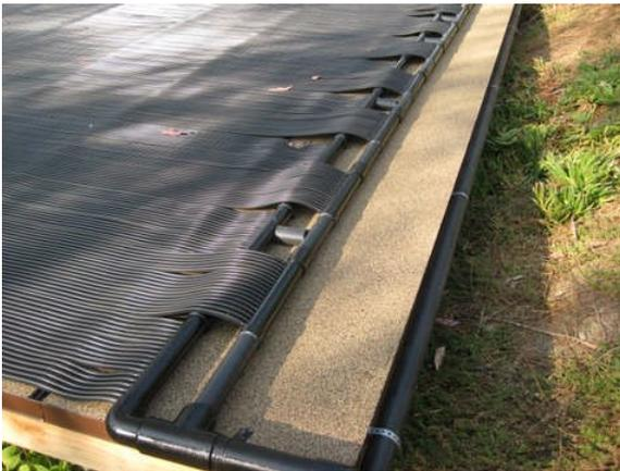
The two rows of headers are teed together at each end. We like to use a street elbow here because it allows the two rows of headers to be closer together. A street elbow is a 90 degree elbow that glues to pipe on one end and right into a fitting on the other.
