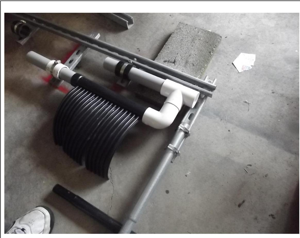
The ballasts are spaced every second header along the top and every 3 feet on the edge bars parallel to the flow.
