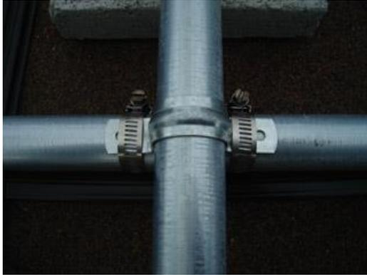
1" 2 hole emt conduit clamps fit the chain link fence top rail perfectly .
