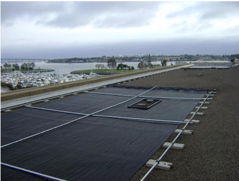
Attach the headers to the top rails with loops of ppa coated ss strap and strap clamps to complete the loops. Make sure the headers can move back and forth with temperature change. Rotate the headers so the fin tube does not abrade on the concrete blocks. Leave room to mount plumbing on the ballasts. Don't commit the position of the ballasts until the last step. Don't apply the construction mastic until the system is plumbed and operating. Then and only then can you be sure of the position.
