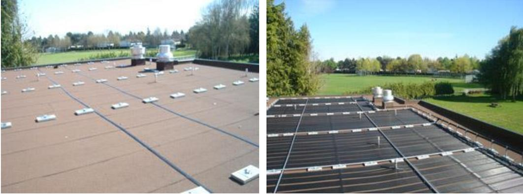
The ends of the glue strips go under the concrete ballasts and then tie off to the framework. Once the job is complete arrange all the fin tubing so it is straight and evenly spaced and then glue the glue strip to the underside of the Powerstrips using construction mastic. Construction mastic takes a while to dry.
