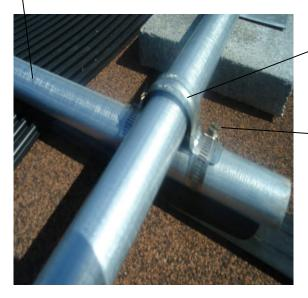
GALVANIZED TWO HOLE CONDUIT CLAMP FOR 1" EMT CONDUIT. NOTE:
